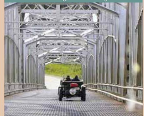
Bentley on Nisutlin Bay Bridge (1957) Photo by L. Gurnsey
